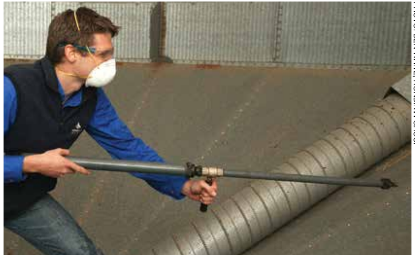
All-over clean: Clean silos, including the silo wall, with air or water to provide a residue-free surface to apply structural treatments.
