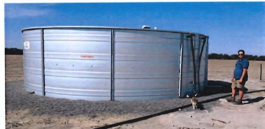
Water is pumped into this header tank (above) from any of the main dams via the piped network. It is then gravity-fed to stock troughs from the tank. The troughs provide a fresh water option for sheep in paddocks with the eight dry / salty dams. Header tank water is also used for spraying and fire fighting purposes.
